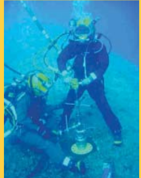
Divers hot tapping a cargo tank on MISSISSINEWA.
